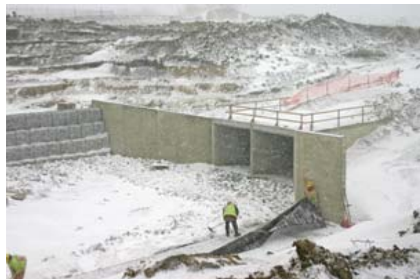
Construction continues on the north airfield landside site
