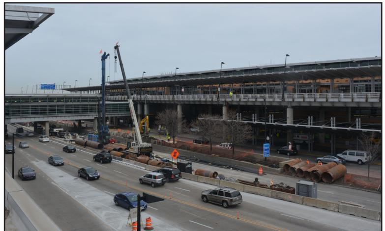
Cicero Avenue and Arrivals traffic flows smoothly around the work area for the bridge. Caisson rigs have been set up on the north side to begin foundation work.
