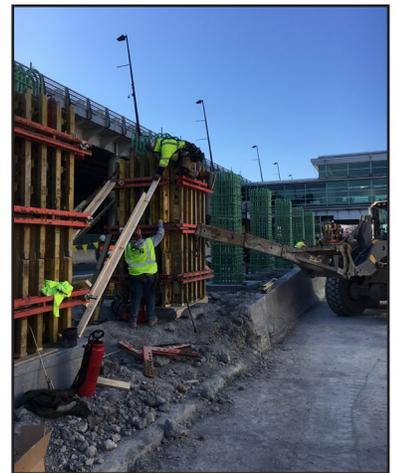
A line of metal forms rise up from Cicero Avenue as crews prepare to set the concrete piers that will support the new bridge as part of the Security Checkpoint Expansion.
